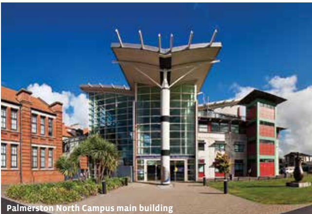
Palmerston North Campus main building
